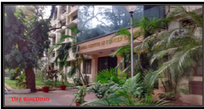
Fig. 4. LIFE building, the place we doing our research
