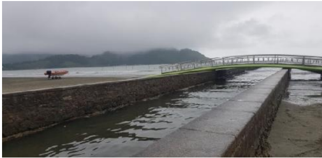
Fig.2: Connection between sea and river to contain Flooding in Santos, Brazil (Author, 2019)
