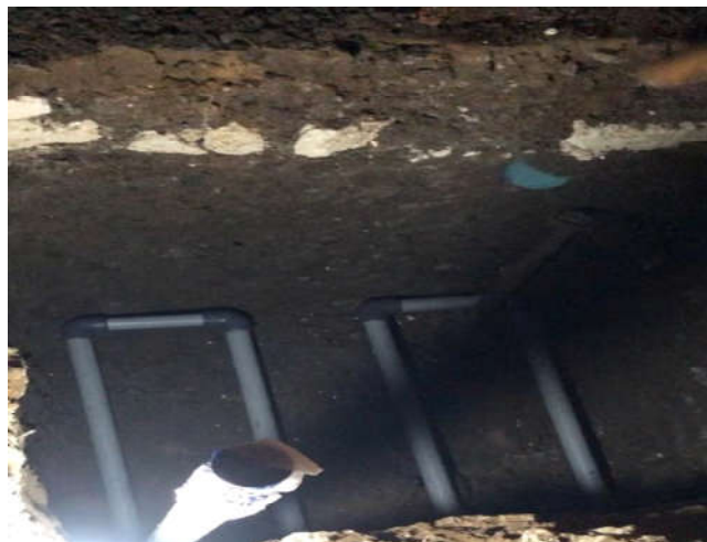
Fig. 5. Installing geothermal pipe
