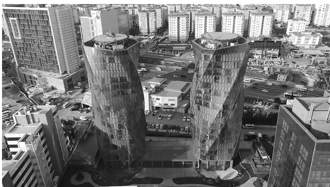
Figure 3. Burgu Towers, the image of the front façade from Seri Street
