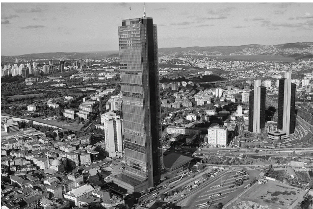
Figure 1. The image showing the location of Sapphire Tower in the urban tissue
