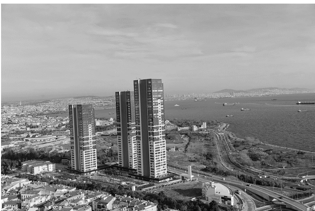
Figure 5. The image showing the location of Onaltıdokuz İstanbul in the urban tissue.
