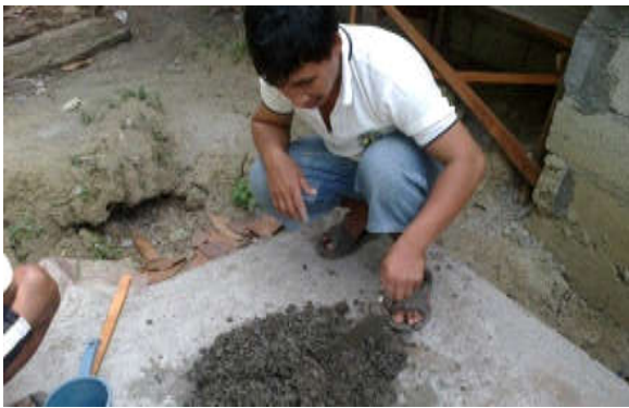
Figure 6. Mixing with Cement
