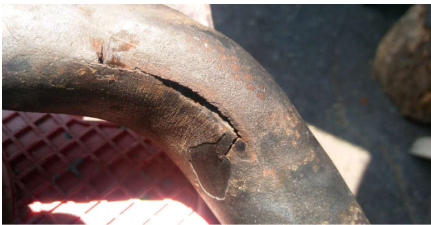
Figure 12. Thermal cracks in exhaust header ( https://www.centuryperformance.com/exhaust-header-heat-wraps-do-not-use.html )
