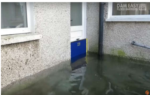
Fig. 2. and 3 Illustrates the arrangement of dam easy barrier (Source: https://www.youtube.com/watch?v=5ZZyYyN2Dcw )
