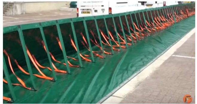
Fig. 8. Illustrates the mechanism of Rapidam flood barrier (Source: https://www.youtube.com/watch?v=5ZZyYyN2Dcw )
