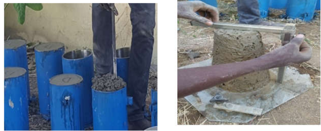
Figure 10. Placement of concrete
