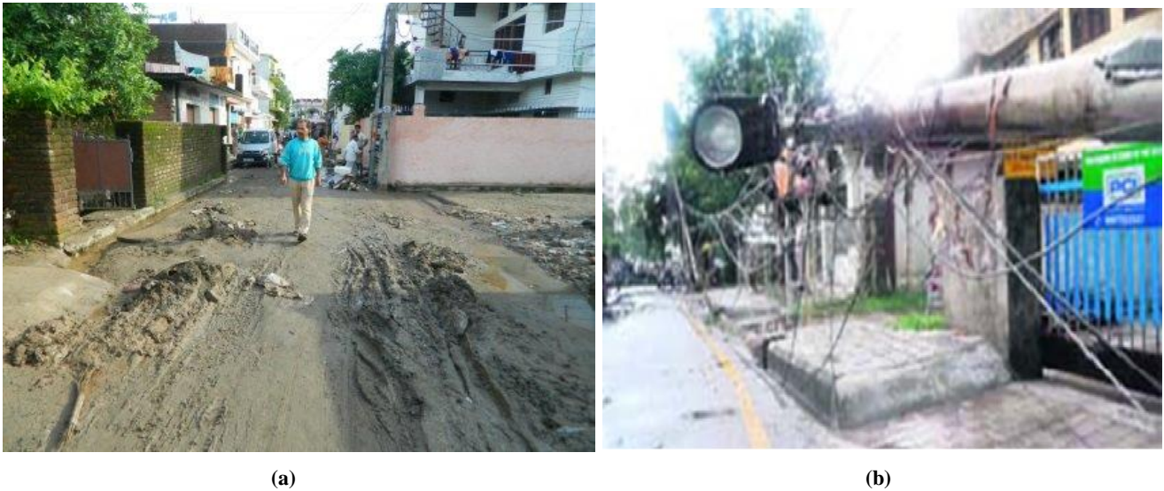
Figure 10. (a) Access road to LDA, filled with mud, June 2013; (b) A view of uprooted electric poles after a dust storm and heavy rain on the Rajpur Road in Dehradun on, June 23, 2010 (The Tribune, Dehradun Plus, 2010b)
